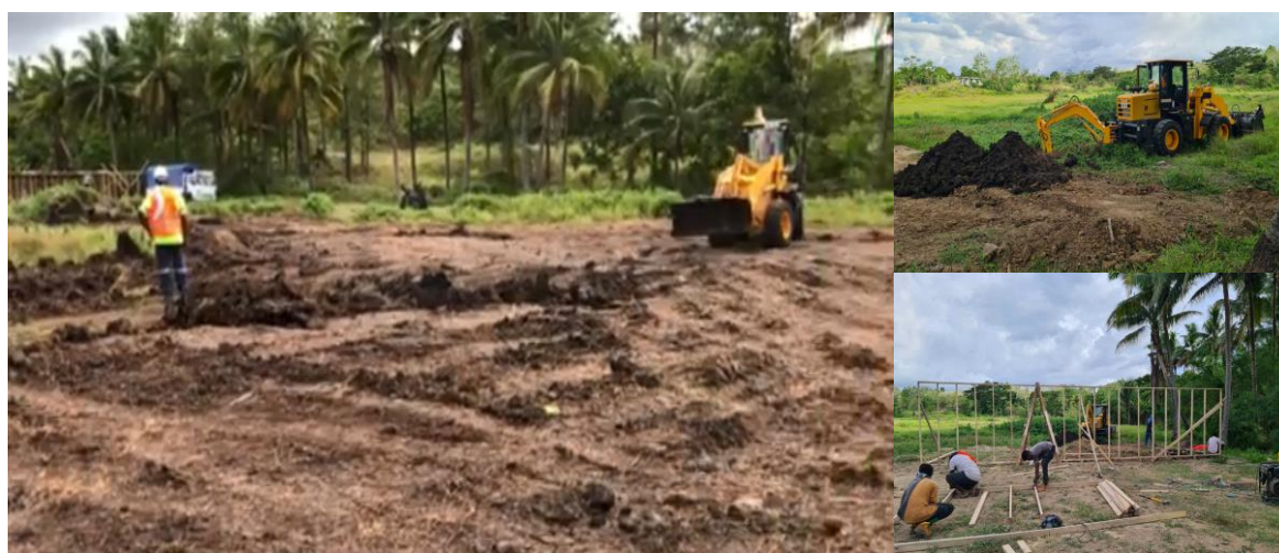
Civil Works, Excavation & Development work have begun in Natabua Teachers Residential Village, Lautoka
