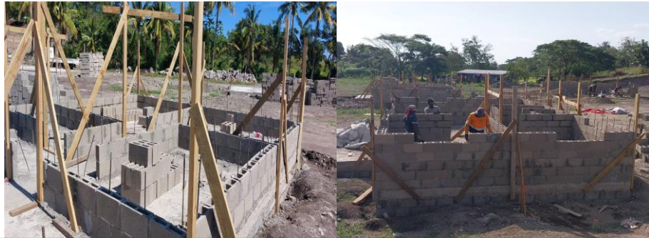
Progress of work at Natabua Residential Teachers Village: 4 x 3 bedrooms and 6 x 2 bedrooms currently constructed.
