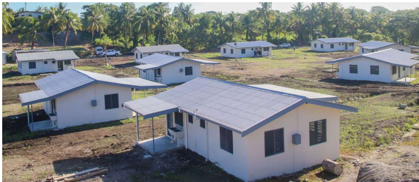
FTA Natabua Teachers village in completion stage
